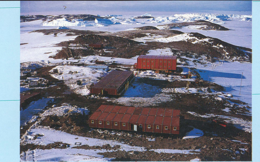
Zhong Shan Station (PRC) Looking west (November 1989) Photo J. Shewin
