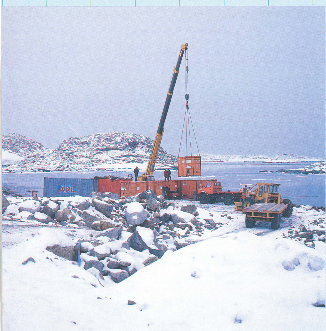
Resupply operations at Casey station. Buntrock Hill lies behind the crane. Part of McMullin Island can be seen in the distance to the right. (Photo: R. Swan)
