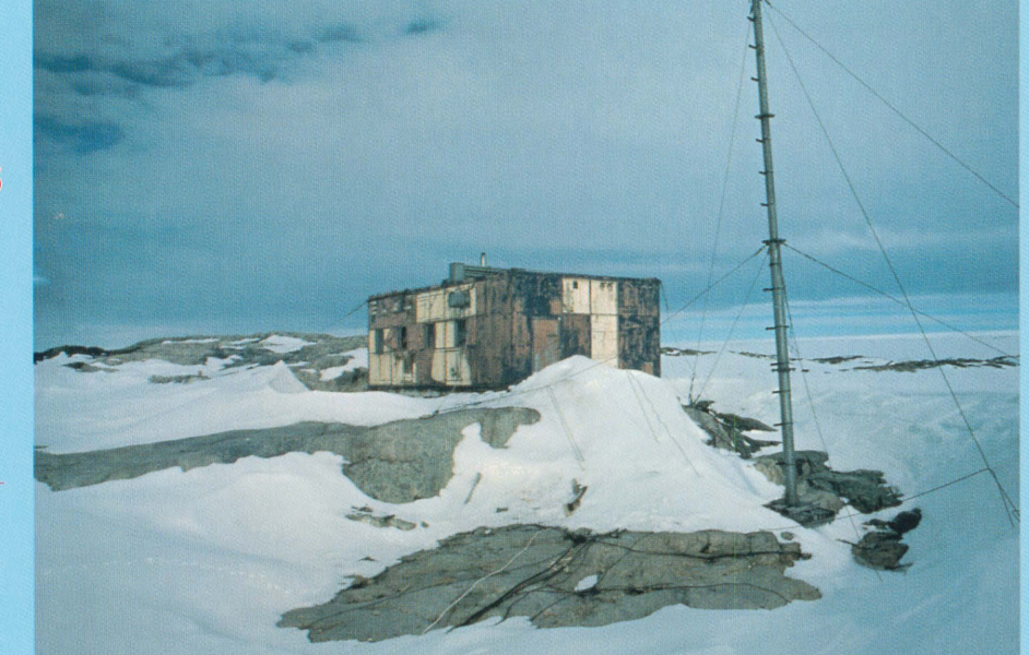
Wilkes Hilton: The old wireless building at Wilkes is a popular field hut. As part of the old Wilkes station, which was abandoned in 1968, this large hut has a rustic charm far removed from the modern feel of the station. (Photography Australian Antarctic Division)
